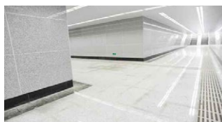
Hotel hallway junctions
