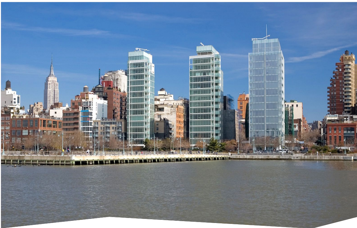
New York's Low-Income Housing Facilities US
